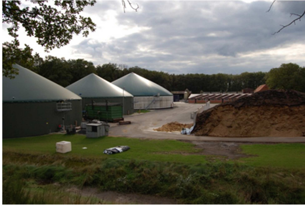
Abb. 12: Biogasanlage in Surwold
